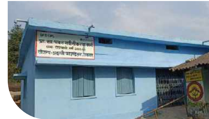
Constructed 8 classrooms and a library in 4 sites - Raigarh (Tamnar), Dahanu, Raipur and Dahej
