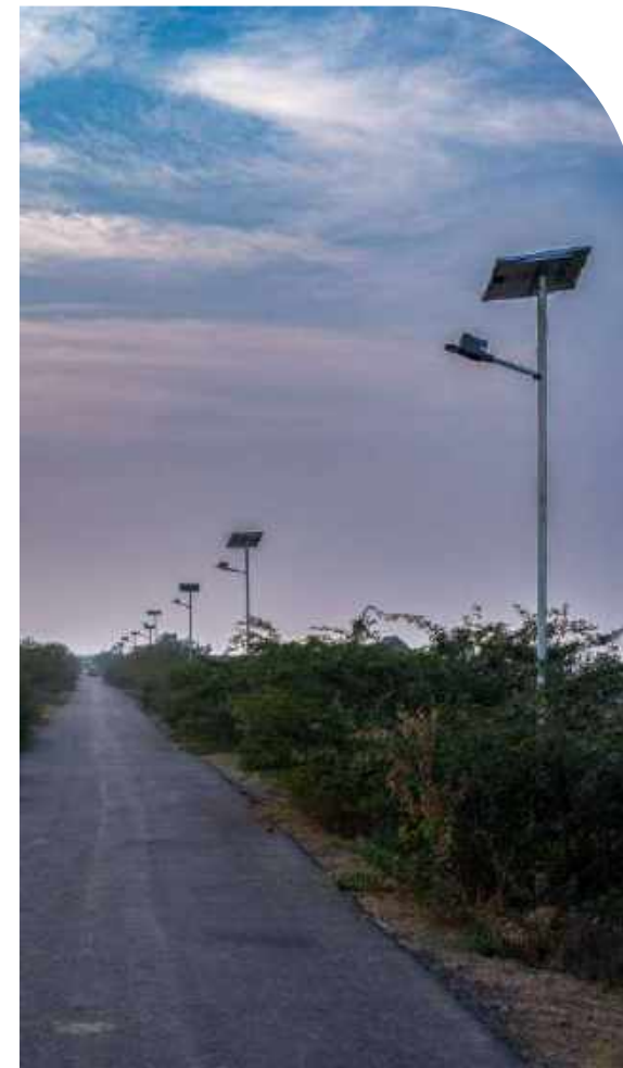
Installed 90 solar streetlights in Dhamra and Raigarh
