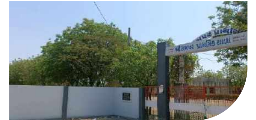
Built 183-meter boundary wall in primary school of Rampar, Mundra
