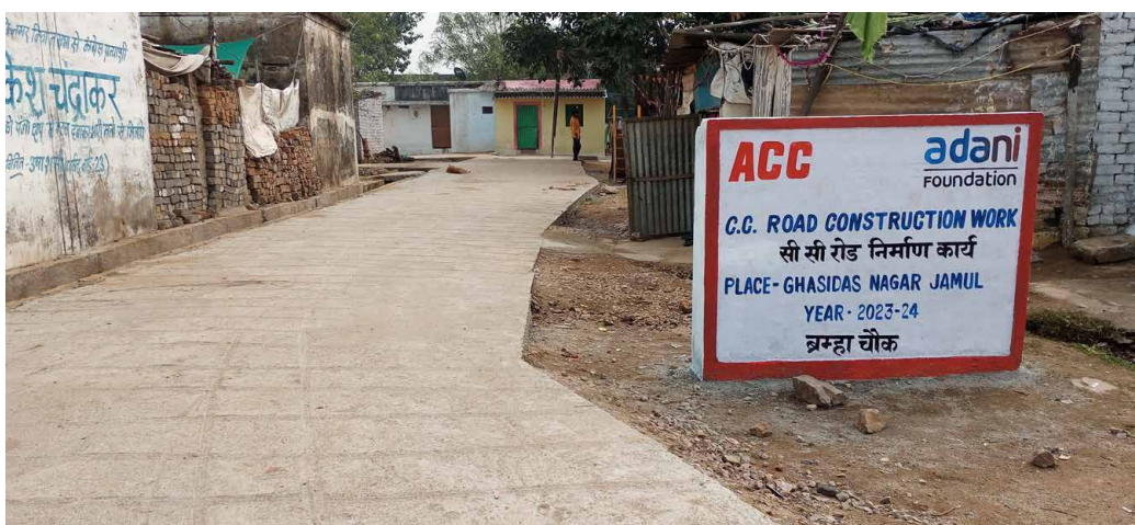
Cement Concrete road - Jamul, Chhattisgarh
