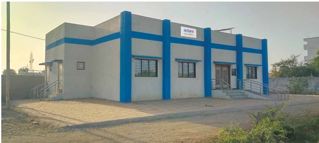
Community Hall - Dahej, Gujarat
