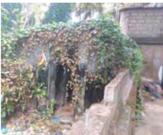
Public Toilet Blocks, Vizhinjam (before)
