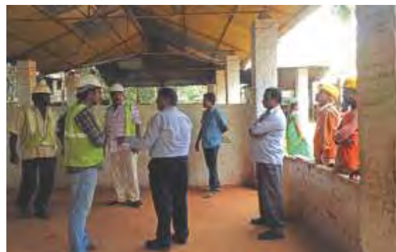
Ongoing Construction of Toilet Block at Ayyankalimaraka UP School, Vizhinjam
