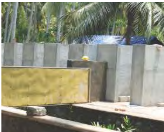
Ongoing Construction of Public Bathing, Vizhinjam
