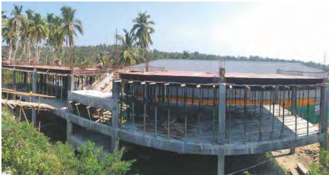
Ongoing Construction at HALP School, Vizhinjam
