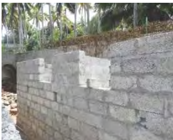
Ongoing Construction of Public Toilet Blocks, Vizhinjam
