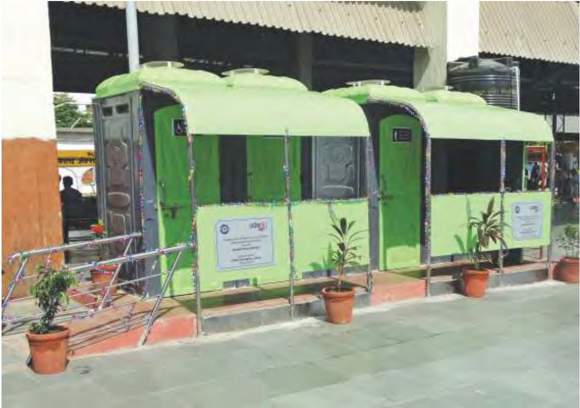
Modular Toilets, Bharuch Railway Station
