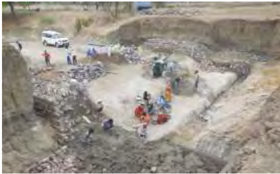
Construction of Anicut, Kawai (before)
