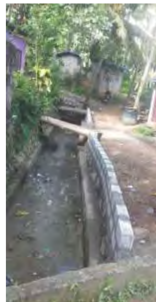
Renovation of Marian Nagar Drain, Vizhinjam (after)
