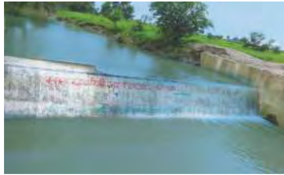
Construction of Anicut, Kawai (after)
