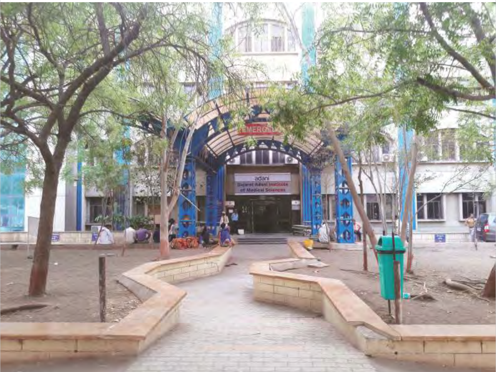
GAIMS-GK General Hospital, Bhuj
