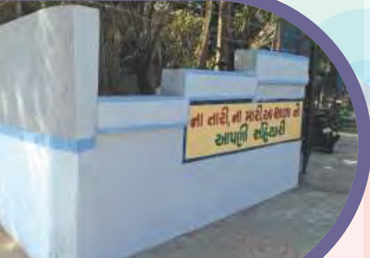
Raising Primary School Compound Wall, Lakhigam
