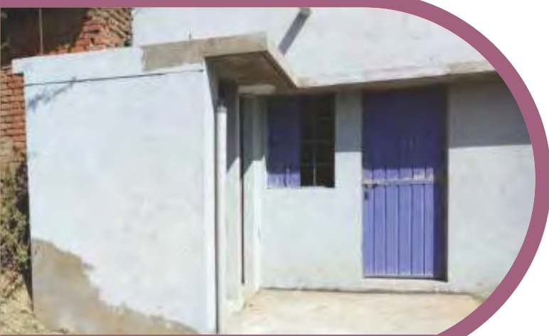
Construction of New Avas, Lakhigam
