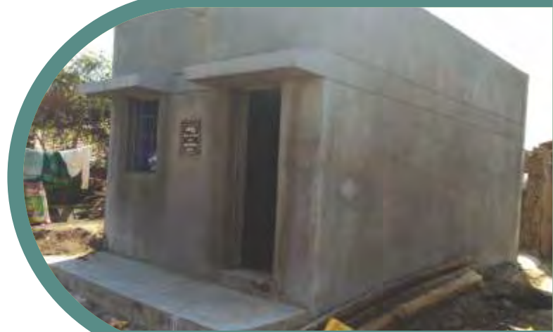
Construction of New Aavas, Lakhigam
