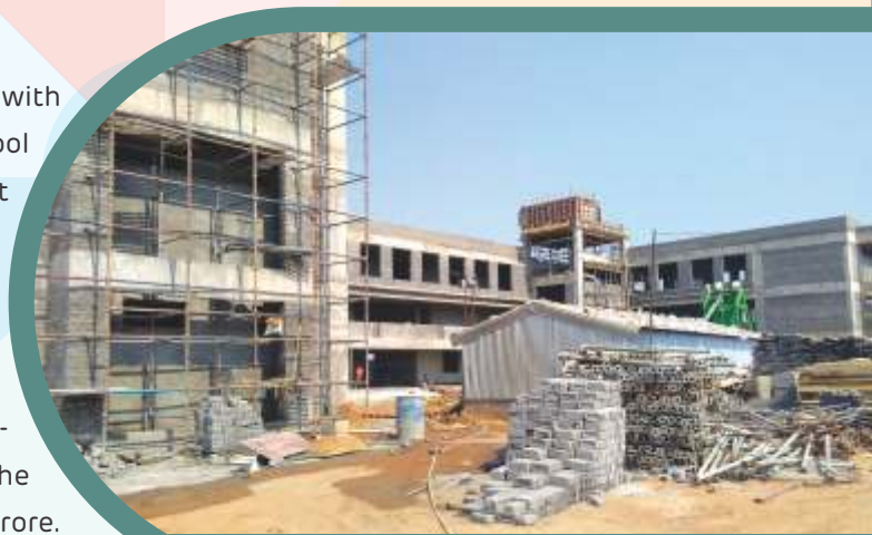
Construction of New Building for Adani-DAV Public School, Dhamra
